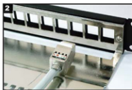
Position the shielded keystone jack for installation.
